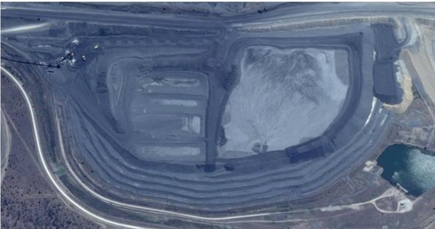
2011 - CDA2 facility exhausted
