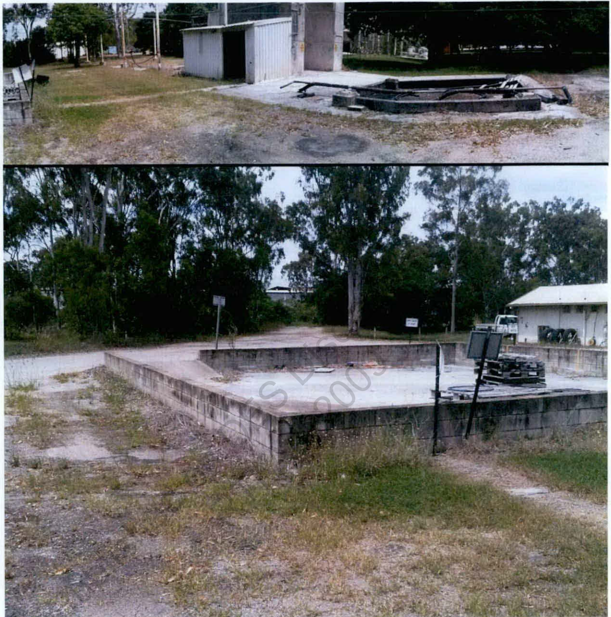
Figure 4-5 (5) Kiln and oil storage area
