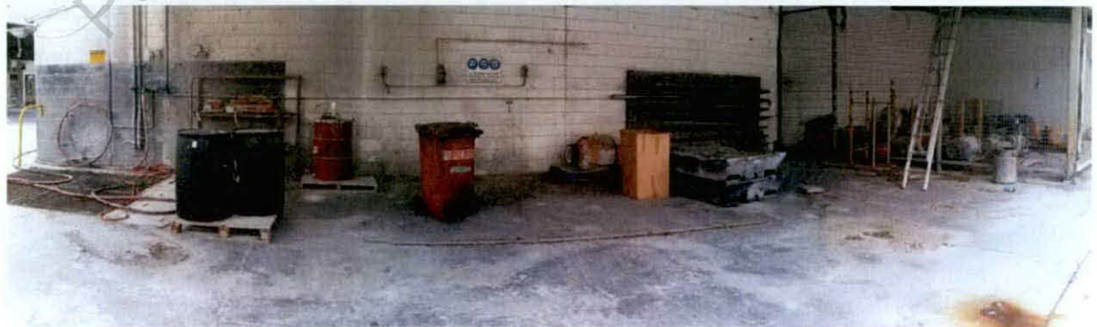
Figure 4-8 (15) Workshop area showing waste oil storage and triple interceptor
