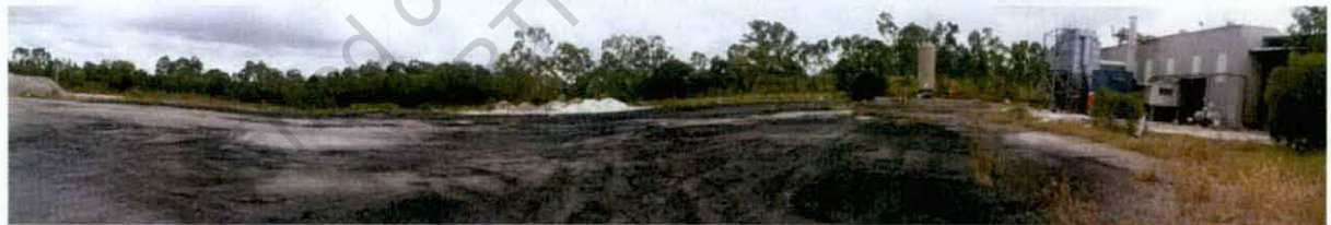
Figure 4-7 (10), (11), (13) Rear of site showing fuel oil and coal storage areas
