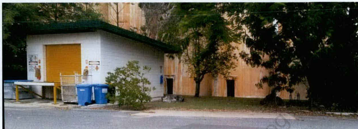
Figure 4-9 (17) Former UST site and oil store.
