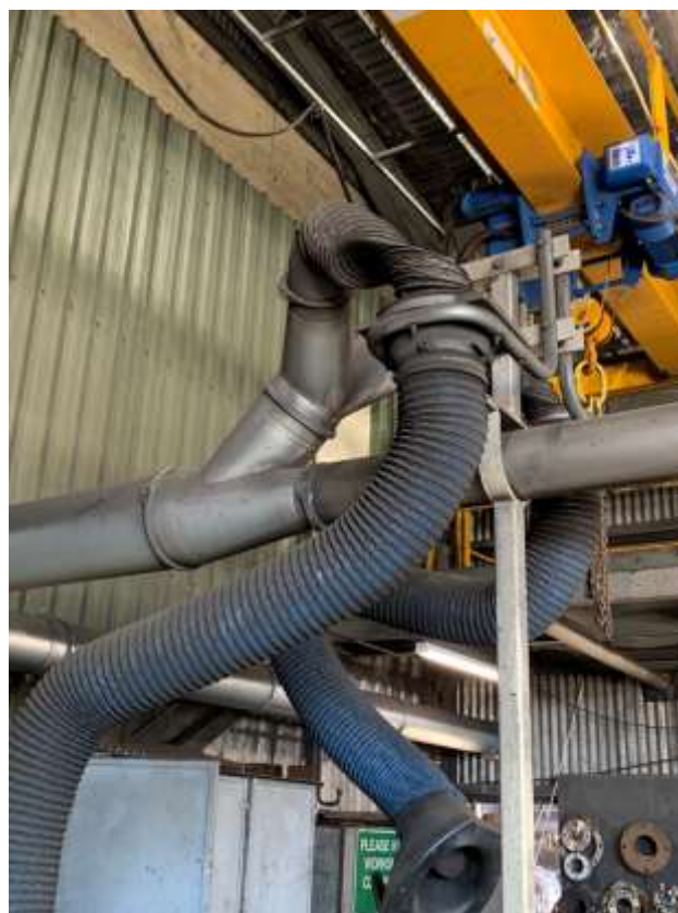
Figure A8: Compromised and poorly maintained LEV systems
