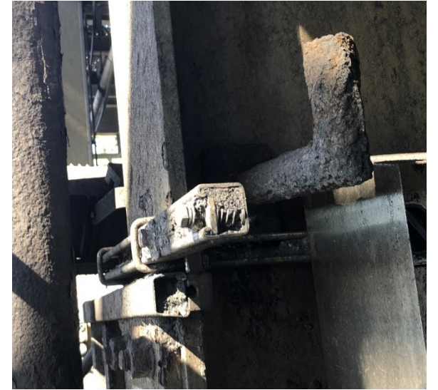
Rusted light fitting bracket
