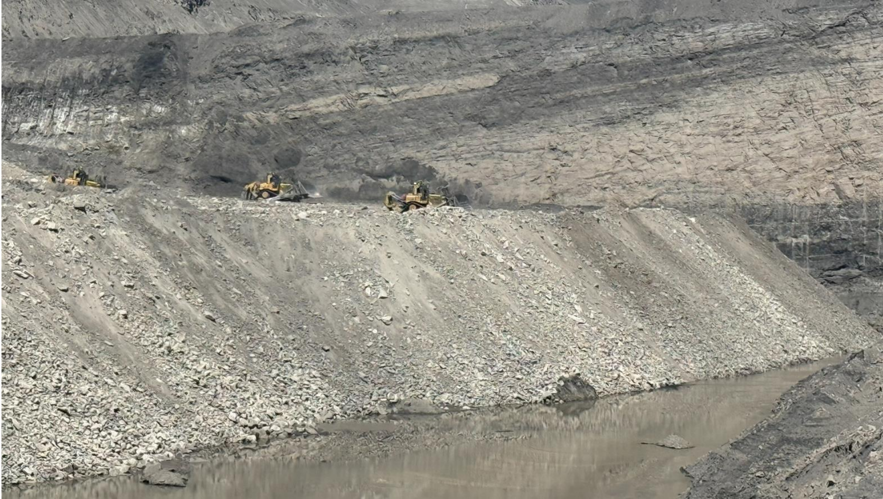
Example Working above water
