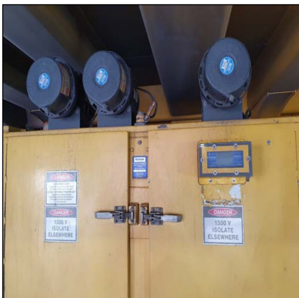
Photos 29 & 30: HEPA Filtration and pressurisation unit fitted to electrical cabinets
