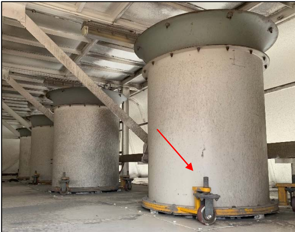
Photo 18: movable intake hood for easy access to dynavanes for cleaning
