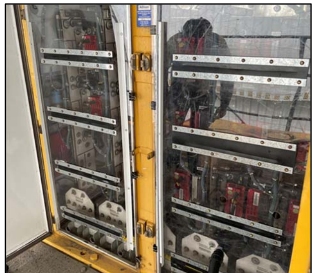
Photo 32: Separation screens between dust generating activity and CMW (electrical cabinets)
