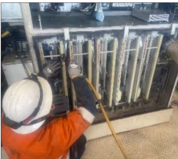
Photo 31: Separation screens between dust generating activity and CMW (electrical cabinets)
