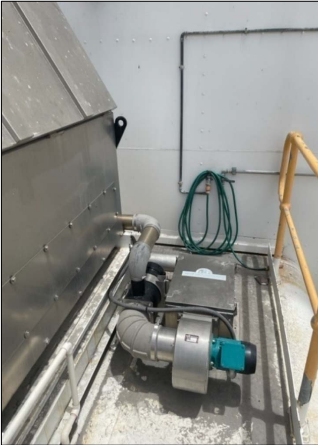
Photo 21: HEPA filtration system for dragline house
