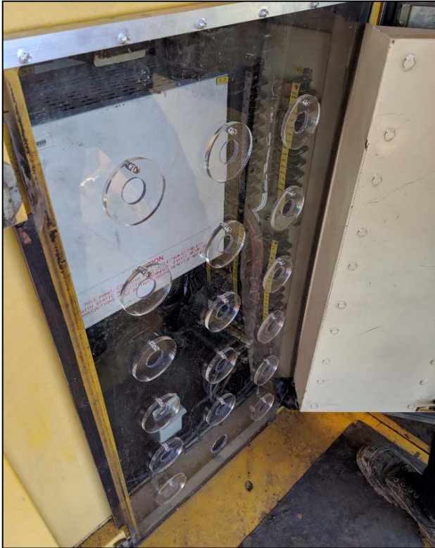
Photo 33: Separation screens between dust generating activity and CMW (electrical cabinets)
